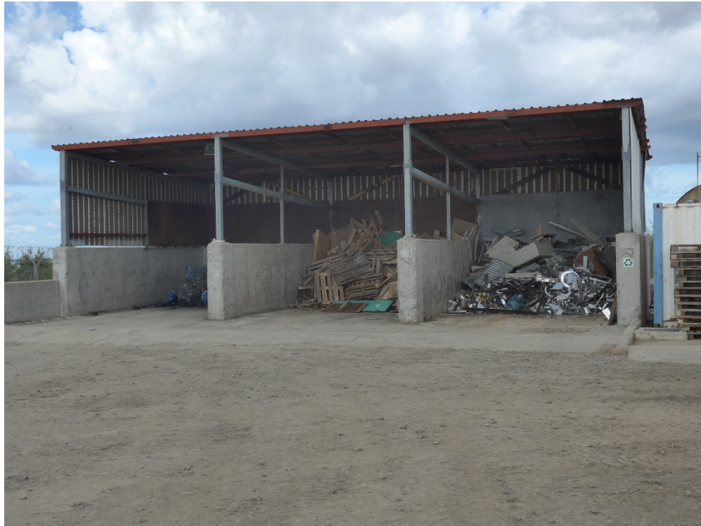
Photo 3. Non-hazardous waste storage at Waste Transit Area
